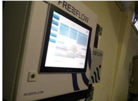
Figure 3 Human Machine Interface (HMI) (5 installed)
