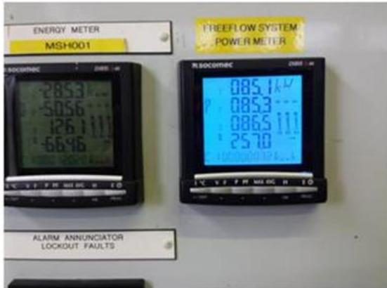
Figure 6 Electrical power metering (26 installed)
