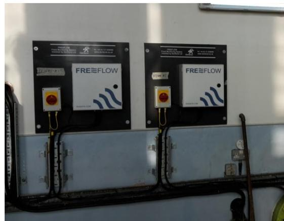
Figure 4 FREEFLOW Data Acquisition Unit (26 installed)
